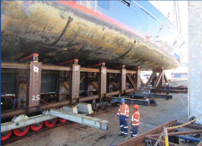
A cradle structure was designed with shaped beams on moving legs contained within fixed uprights and a jacking structure provided for hydraulic jacks. The shaped beams were fitted to the hull shape using a laser scan of the hull (from an earlier haul out). The vessel was successfully jacked (by Rich Rigging) using 14 synchronised single acting jacks.
